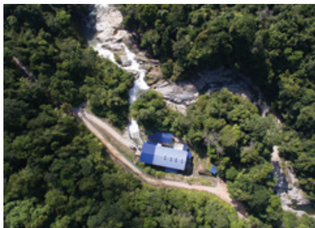
Amcorp Perting Hydro 6MW, Bentong, Pahang.
