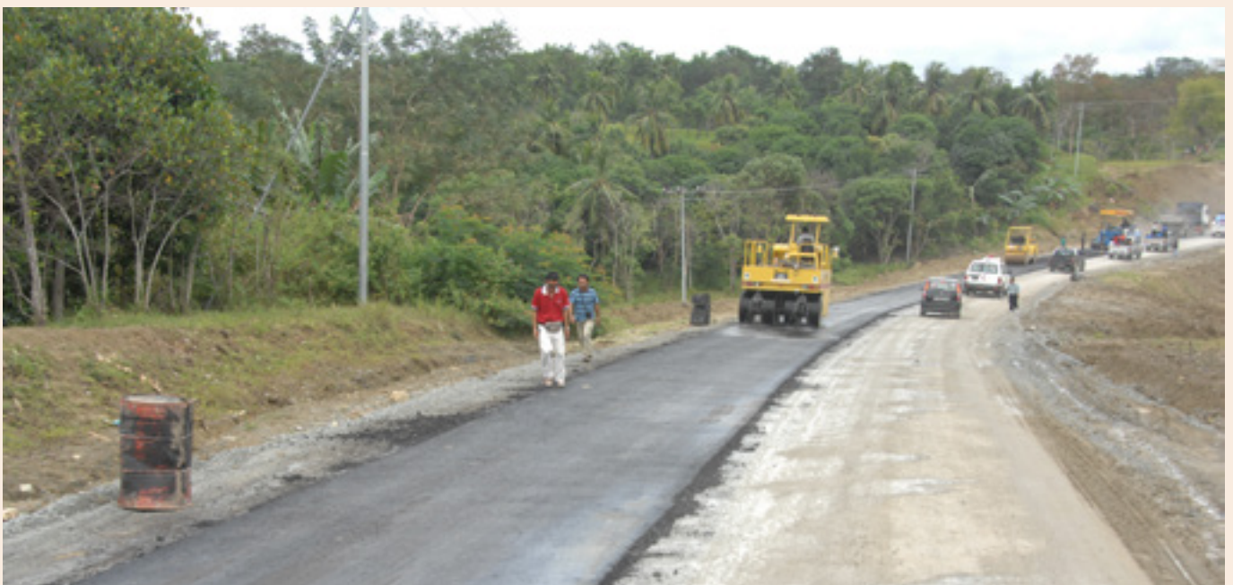
Construction in progress for rural road development.
