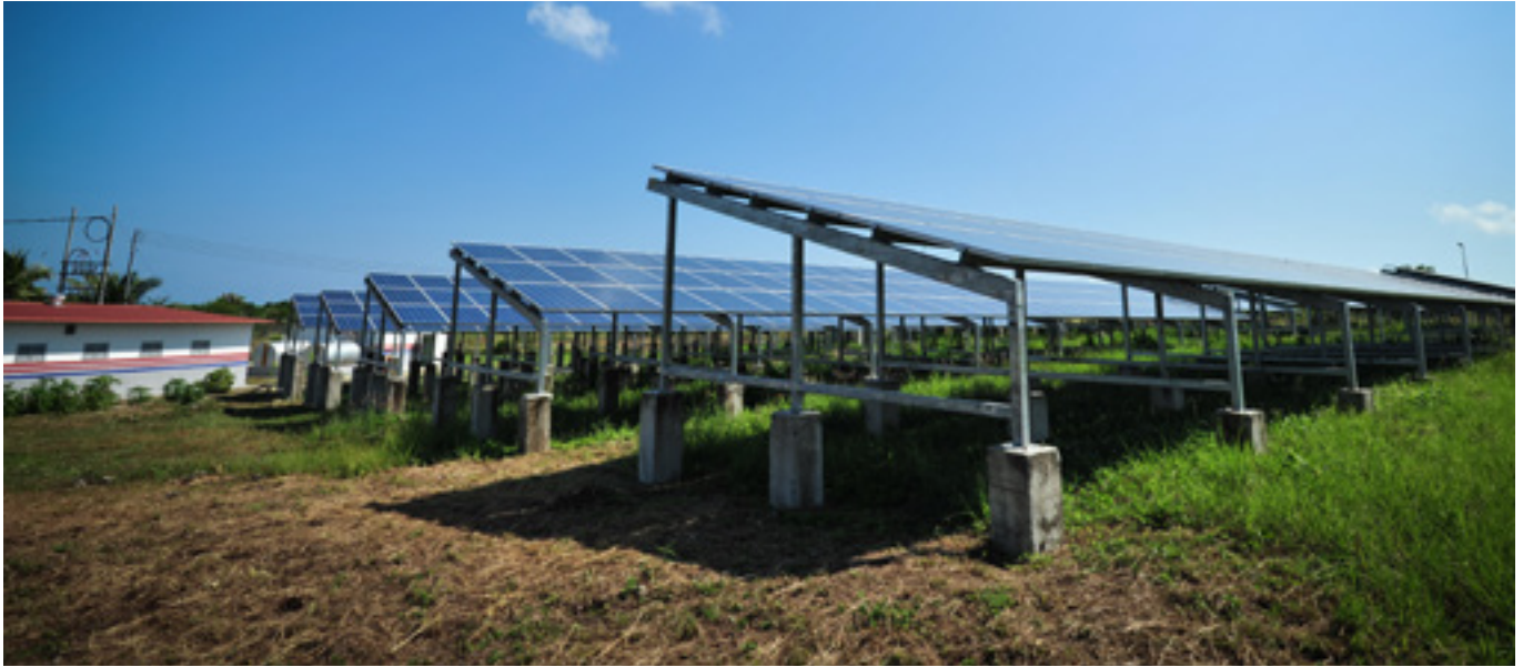
Solar hybrid stations under Program Bekalan Elektrik Luar Bandar.
