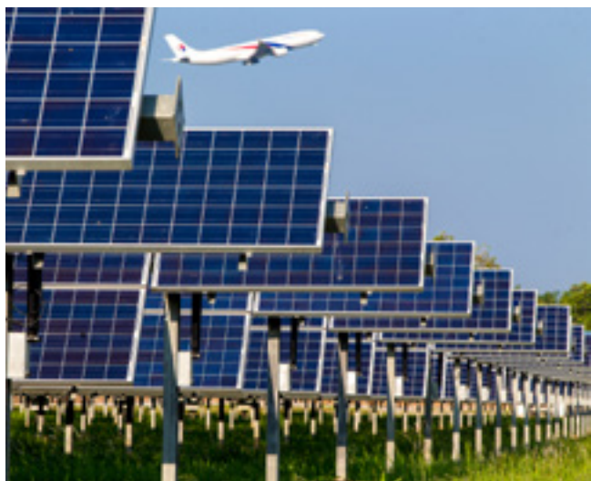
Fortune 11 Sdn Bhd's 5 MW solar farm in Sepang, Selangor.
