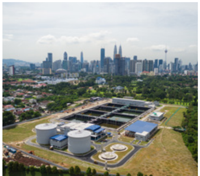
The Bunus Sewage Treatment Plant is part of the larger effort of improving river water quality at Sungai Bunus.
