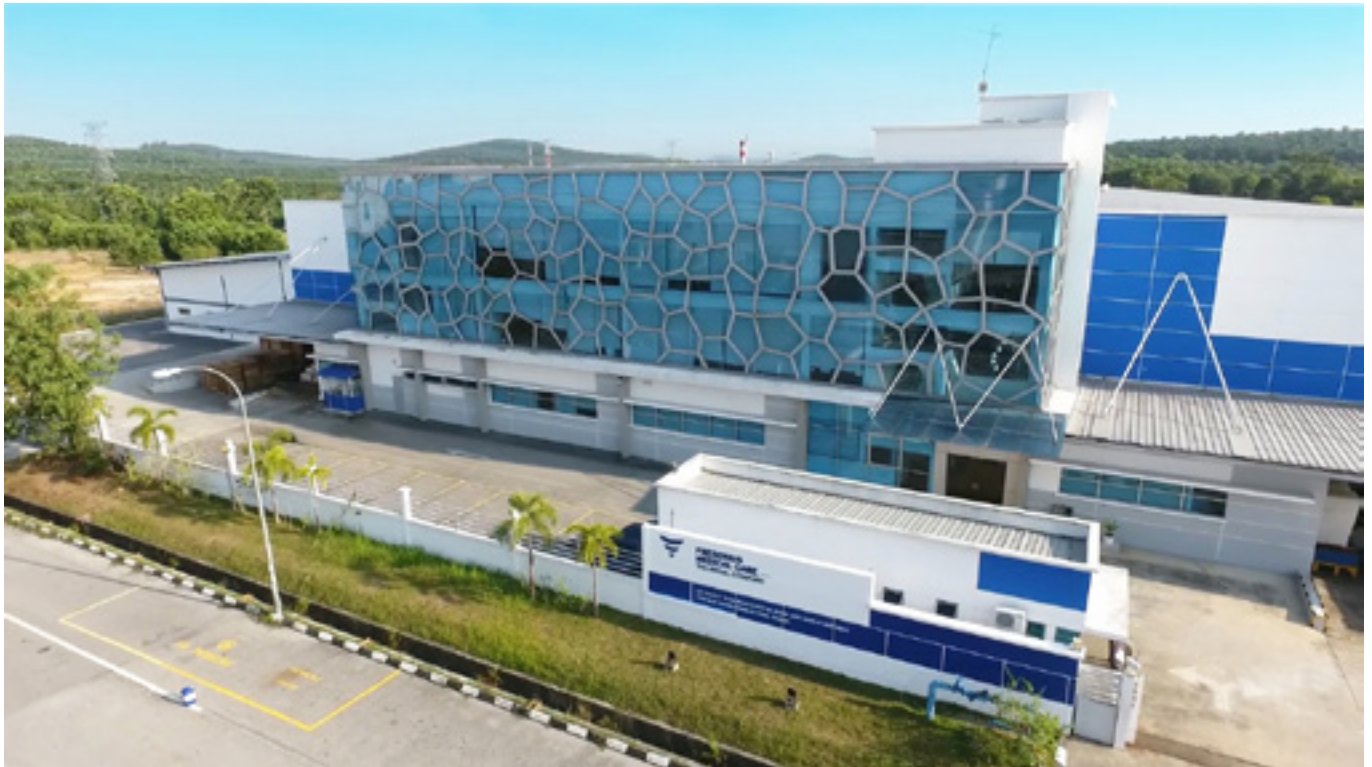
Fresenius Medical Care Sdn Bhd (FME) regional manufacturing facility in Bandar Enstek.
