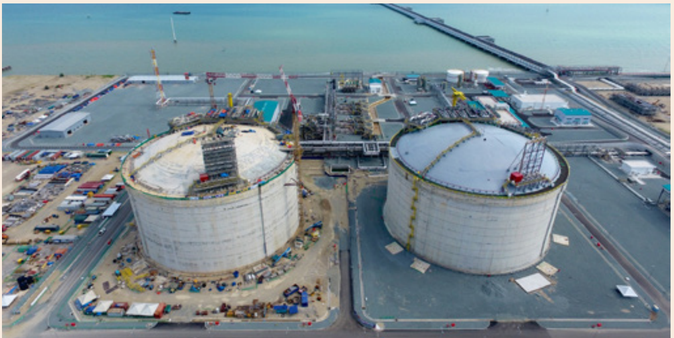
Regasification Terminal 2 (RGT2) in Pengerang started commercial operations at the end of 2017.
